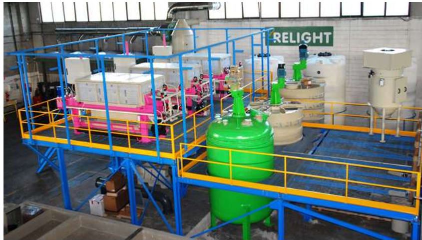
Fig. 4 Fixed plant under construction from Hydroweee Demo Project.
